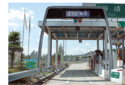
ETCゲート [電波吸収体 (導電性ポリエチレンフォーム)] ETC gate [radio wave absorber (conductive polyethylene foam)]
